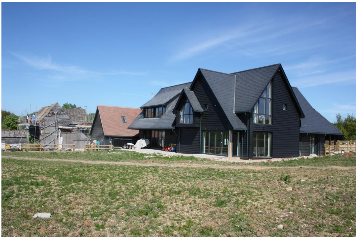
Fig. 4 – a new house at Noaks Cross, Great Braxted. A legal agreement between the owner and the Council requires the repair of the adjacent barn within one year of the completion of the house. The repair of the barn is currently underway.
