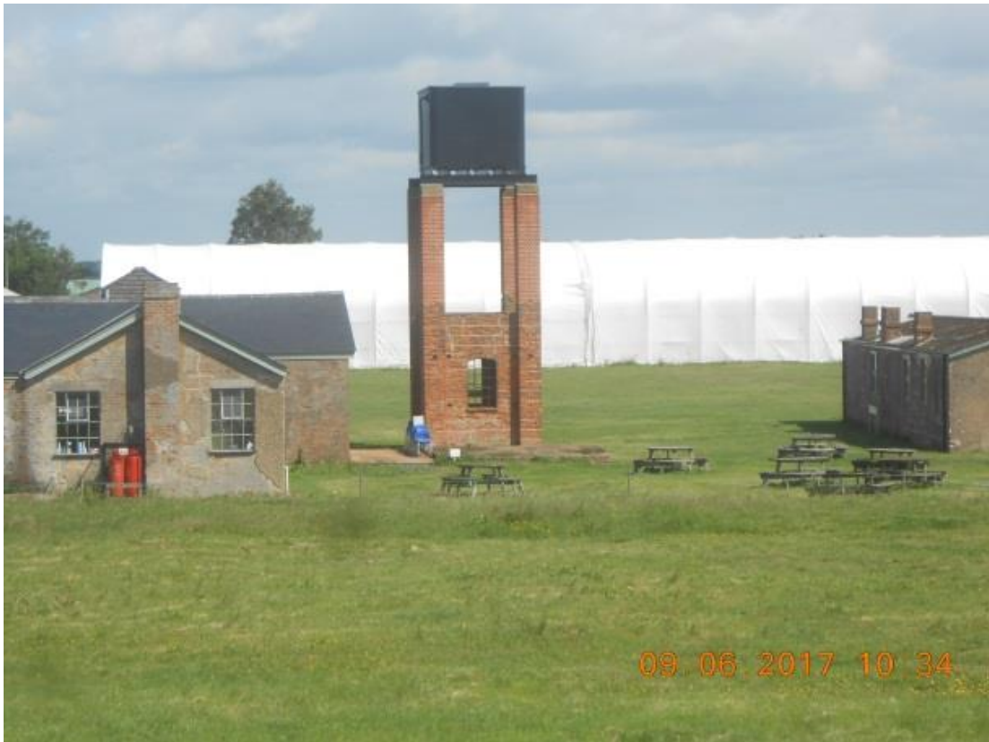
Fig. 5 – The Water Tower at Stow Maries Aerodrome was repaired in 2017
